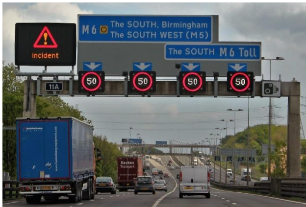
Figure 6: Variable Speed Limit Display in a Motorway in United Kingdom
