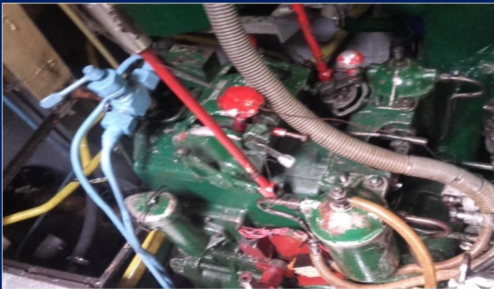
VISIBLE LIGHT IMAGE OF MARINE GEAR BOX
