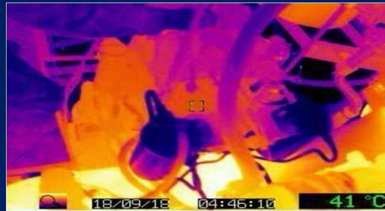
THERMAL IMAGE OF MARINE GEAR BOX
