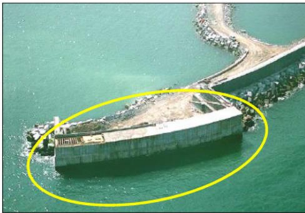
Figure 3: Multi-chamber OWC plant integrated into a breakwater, Spain
