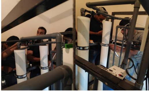
Figure 10: Modifying the plumbing arrangement
