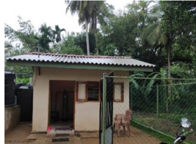
Figure 4: BWRO Facility building
