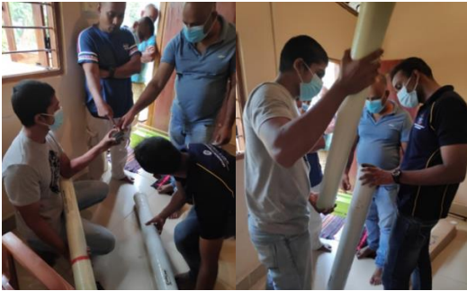
Figure 5: Inserting the new BWRO membrane to the pressure vessel
