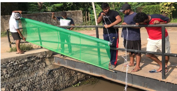
Figure 5. Boom used in the prototype
