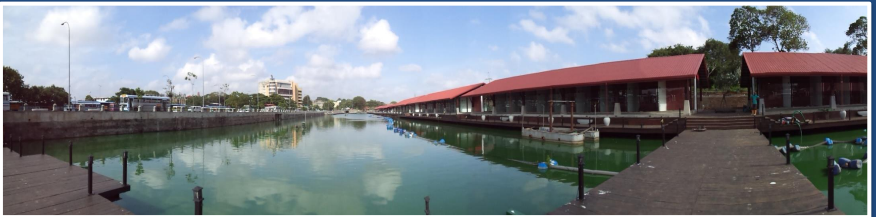
Construction of a new shopping complex at Bastian Mawatha, Colombo
