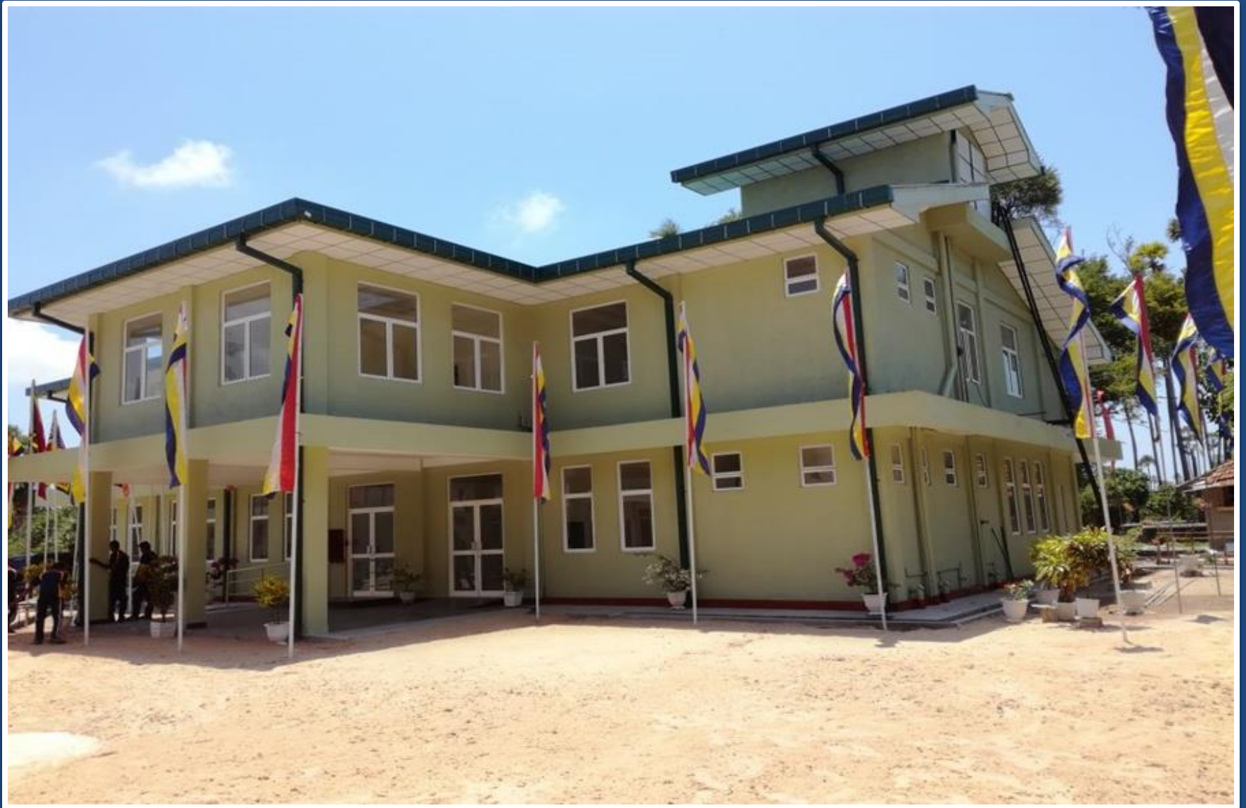
Construction of Divisional Medical Officer's Office - Maruthankeni
