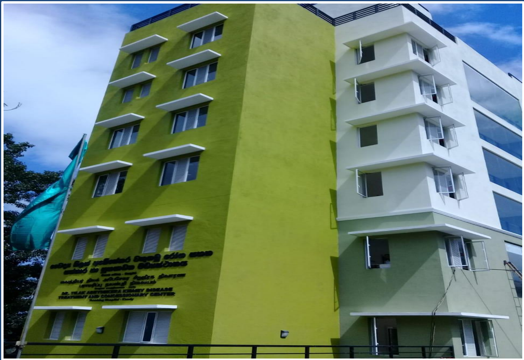
Construction of Kidney Hospital at Kandy
