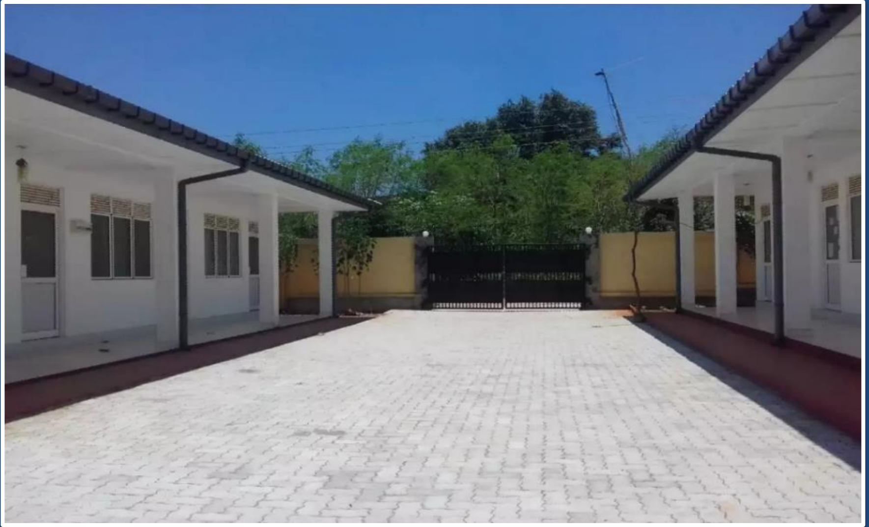
Construction of Kidney Research Center at Medawachchiya
