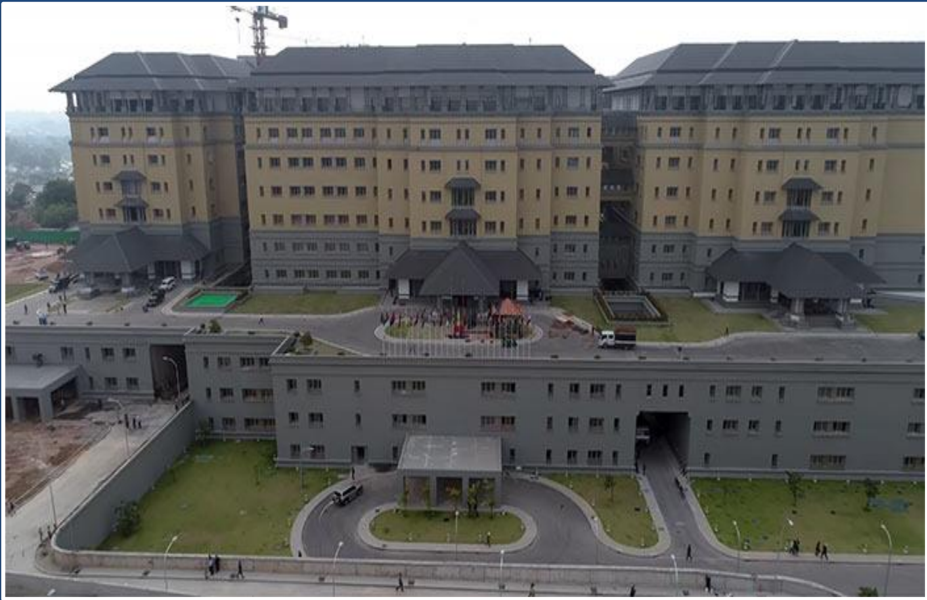
Construction of Defence Headquarters Complex, Akuregoda
