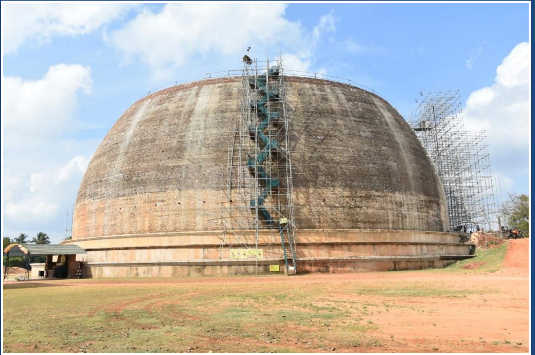
Construction of Sandahiru Seya
