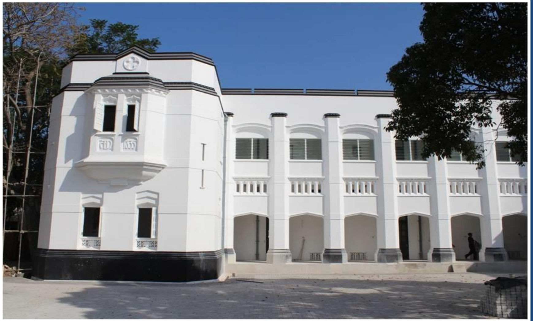
Renovation of Mathematics Section Building of the University of Colombo
