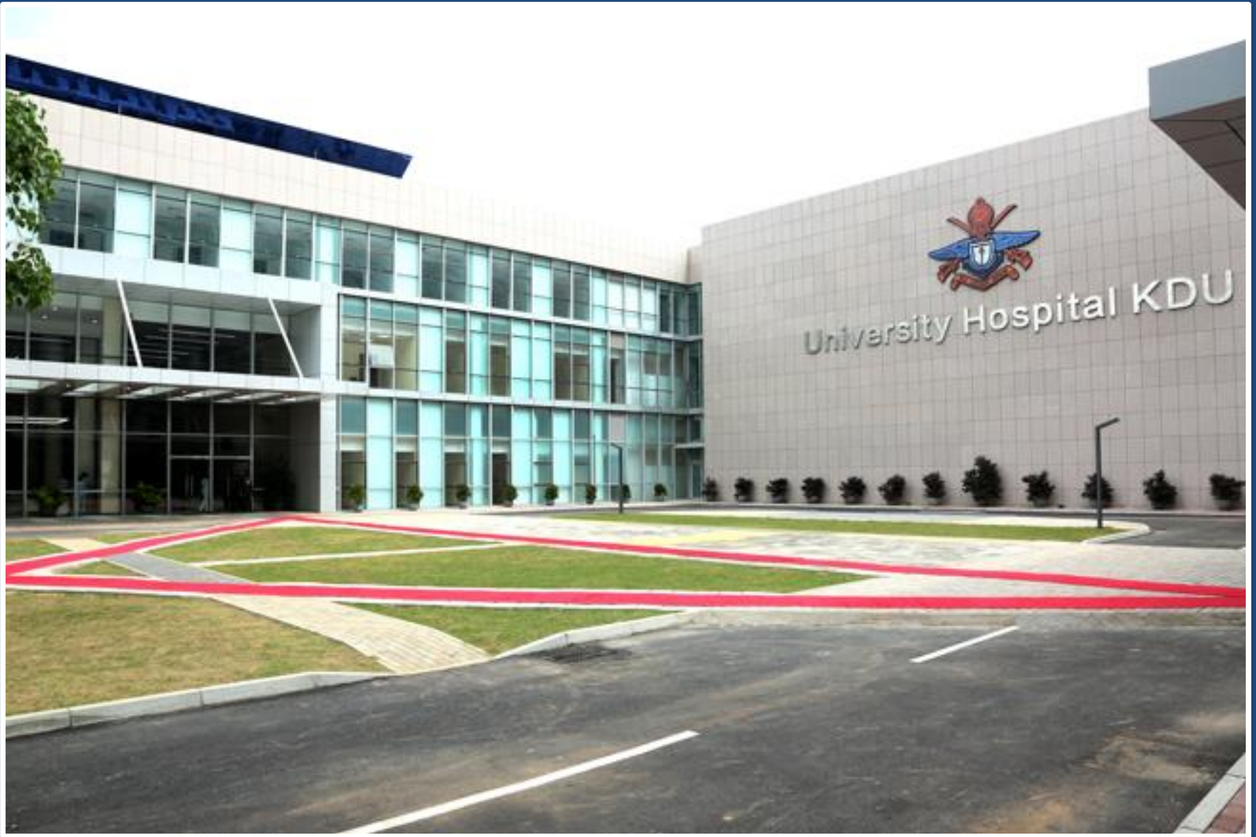
Construction of University Hospital KDU
