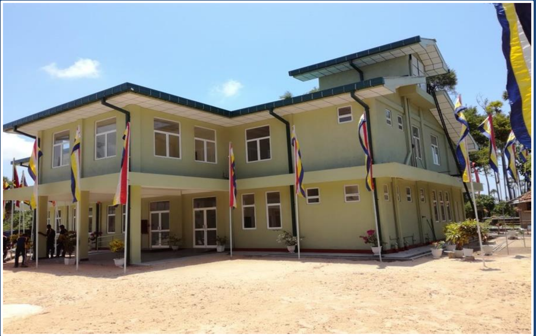
Construction of OPD at Kytes
