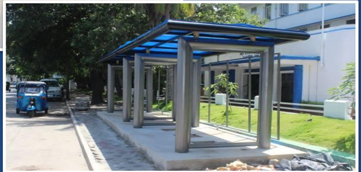
Construction of 57 x bus stops in Colombo city
